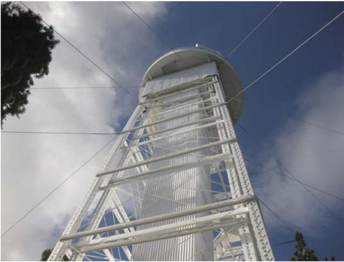
This was a fire hazard and the crude building was replaced with an aluminum shell in 1911. The spectrograph is located in a 15-foot pit. Many important observations were made with the Snow telescope and its instruments but tests soon indicated that a vertical construction would avoid some of the problems associated with heat from the sunlit ground near the mirrors. Shortly after going into operation in 1904, plans were started for building the 60-foot Solar Tower.
