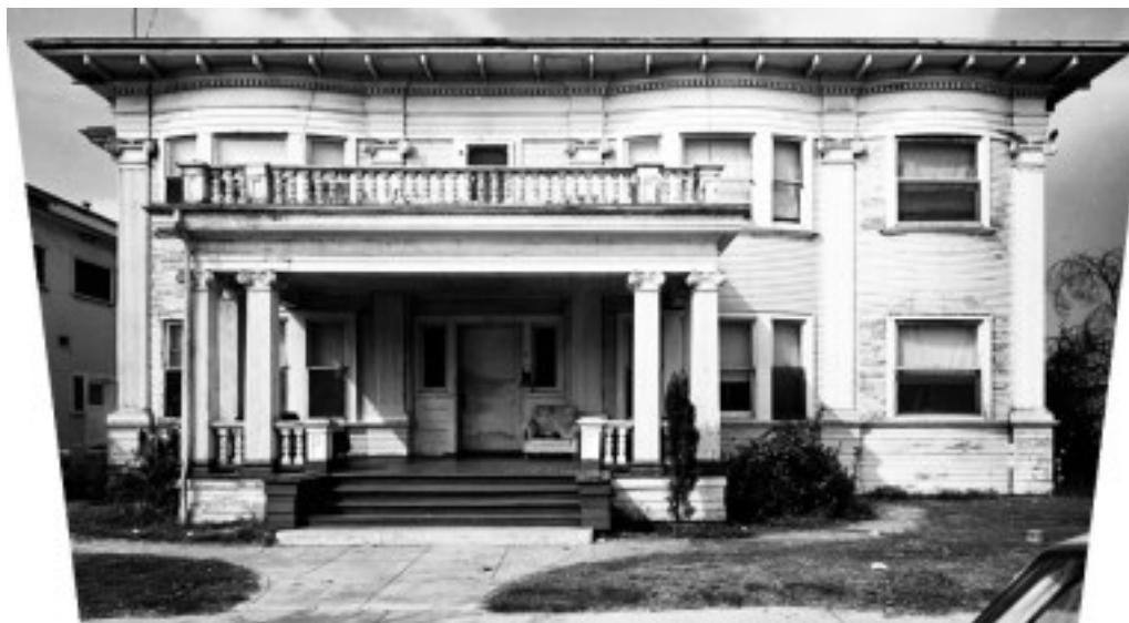
Fig. 2. A victim of urban renewal, the Greek Revival home of Dr. Herbert M. Bush, 2627 South Hoover Street, as it appeared in September, 1977, shortly before demolition. Originally equipped with a rooftop observatory, it was a popular rendezvous for local amateur astronomers. (Image: Los Angeles Public Library, William Reagh Collection.).
